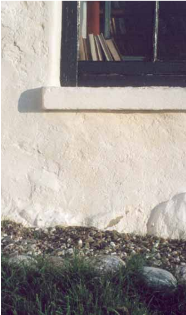
Lime washed wall with French drain to the base of the wall at Termon House, Donegal, conserved by the Irish Landmark Trust.
