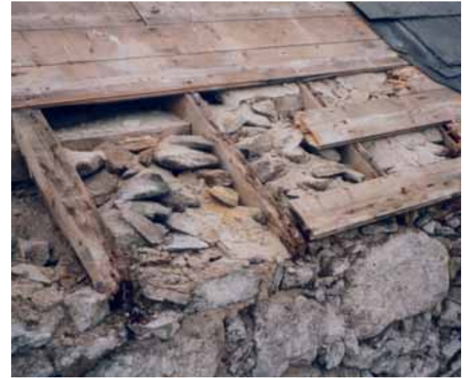
Above: Timber rafters built into top of wall showing degeneration over time due to failure of slate covering at Termon House, prior to conservation.
