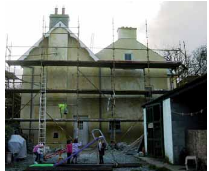
Below: Grant-assisted project showing new lime wash over recently applied lime render to the house exterior at Gower, County Clare.
