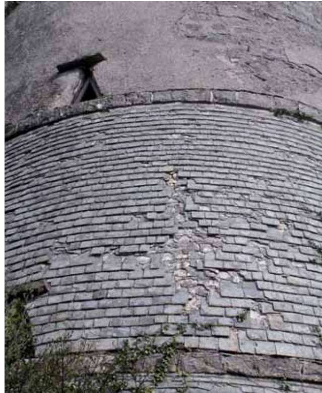
Vertical slate detail set into lime at the Wonderful Barn, near Leixlip.
