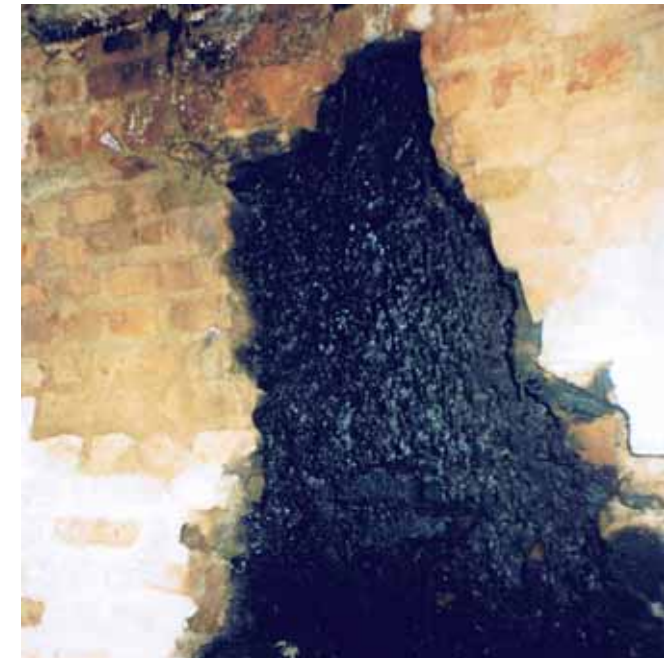
Disintegrating chimney flue due to damp ingress and lack of use.
