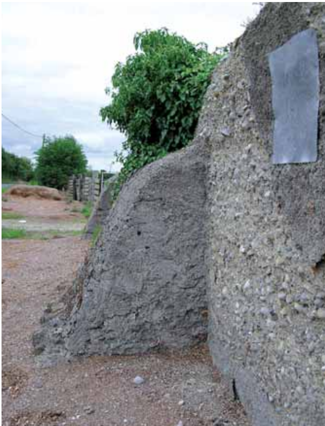
Mud boundary wall with buttress near Nurney.
