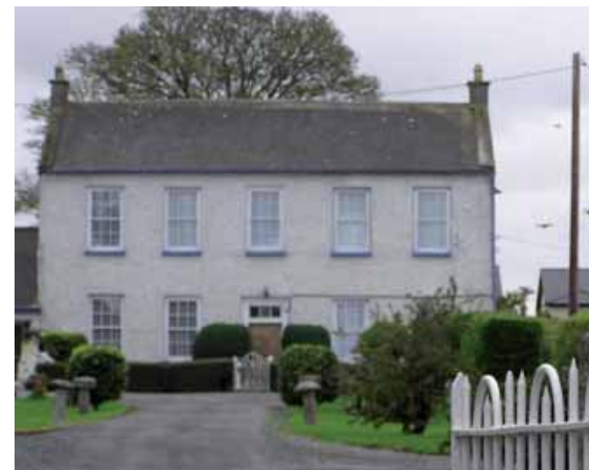
Beside Jigginstown House, a farmhouse with exposed eighteenth century sash windows
