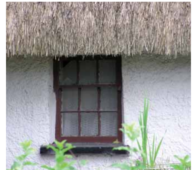
Authentic details including historic sash window, lime rendered walls and overhanging thatched roof.
