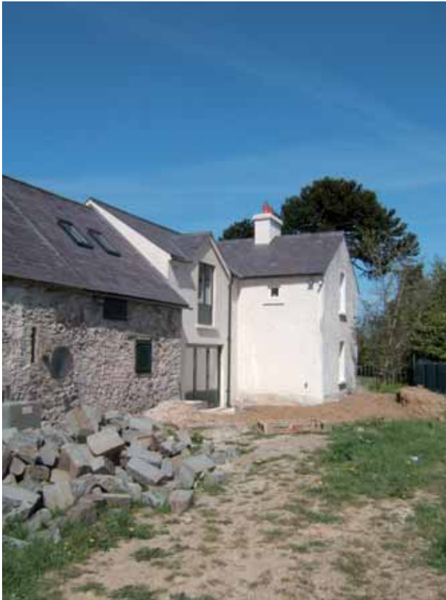
Above: Side view taken from the kitchen garden, showing the infill addition recessed to differentiate it from the original structure. Right: The kitchen, the heart of the house.
