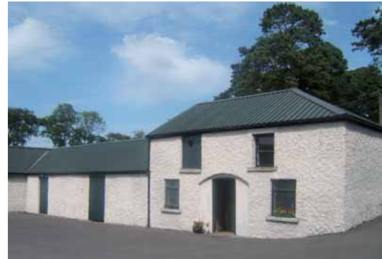
Bottom left: Preservation of thatched structure near Nurney, temporarily protected with plastic-wrapped roof. Above: Significant road-fronting farm complex at Halverstown cross-roads preserved with corrugated metal roofs.
